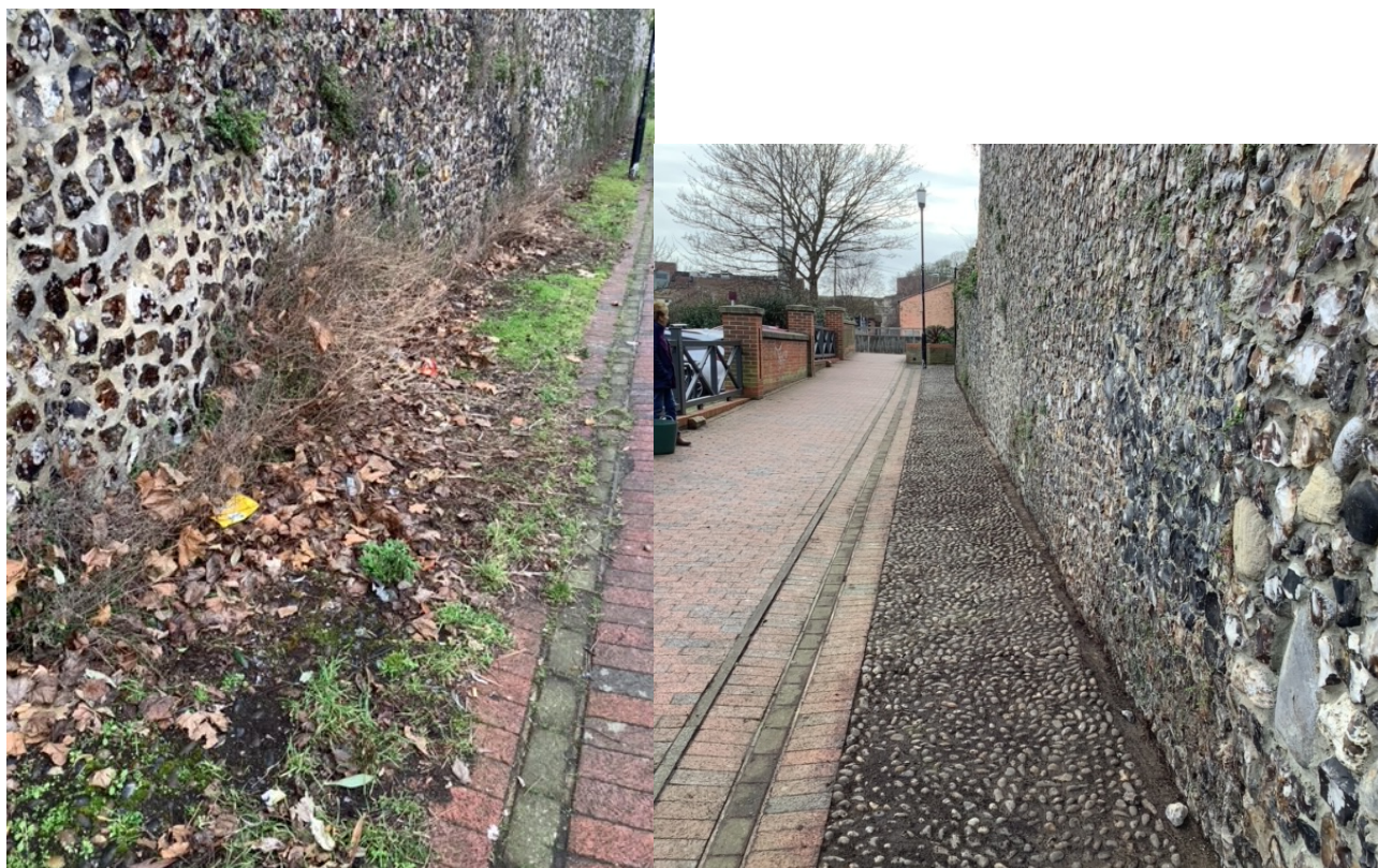
Town Wall near Sainsbury Car park before and after cleaning and weeding
