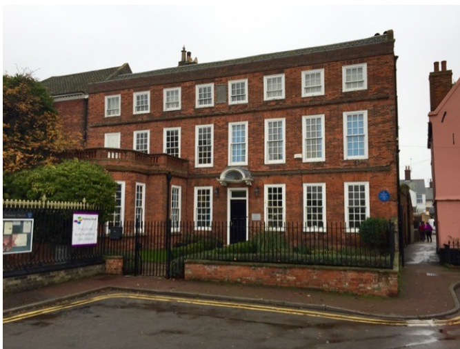
Old Rectory / Credit: H Sturzaker
