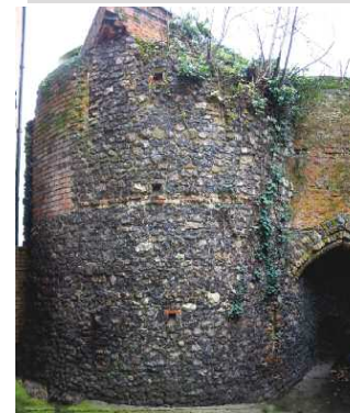
North side of Shave's Tower, as seen from behind the Nurses Home. Right of tower shows the squinch arch.
