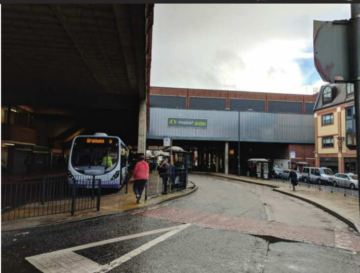
The dismal area of the Market Gates Bus Station
