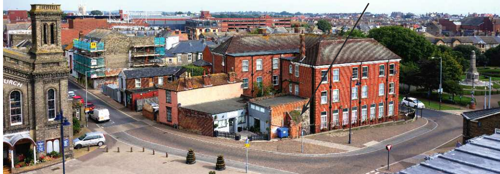
Aerial view of Deneside, illustrating the spacious area for the possibility of New Gate to be re-erected.
