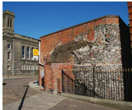
South side of Shave's Tower, which would need to be disentangled from the modern brickwork building.
